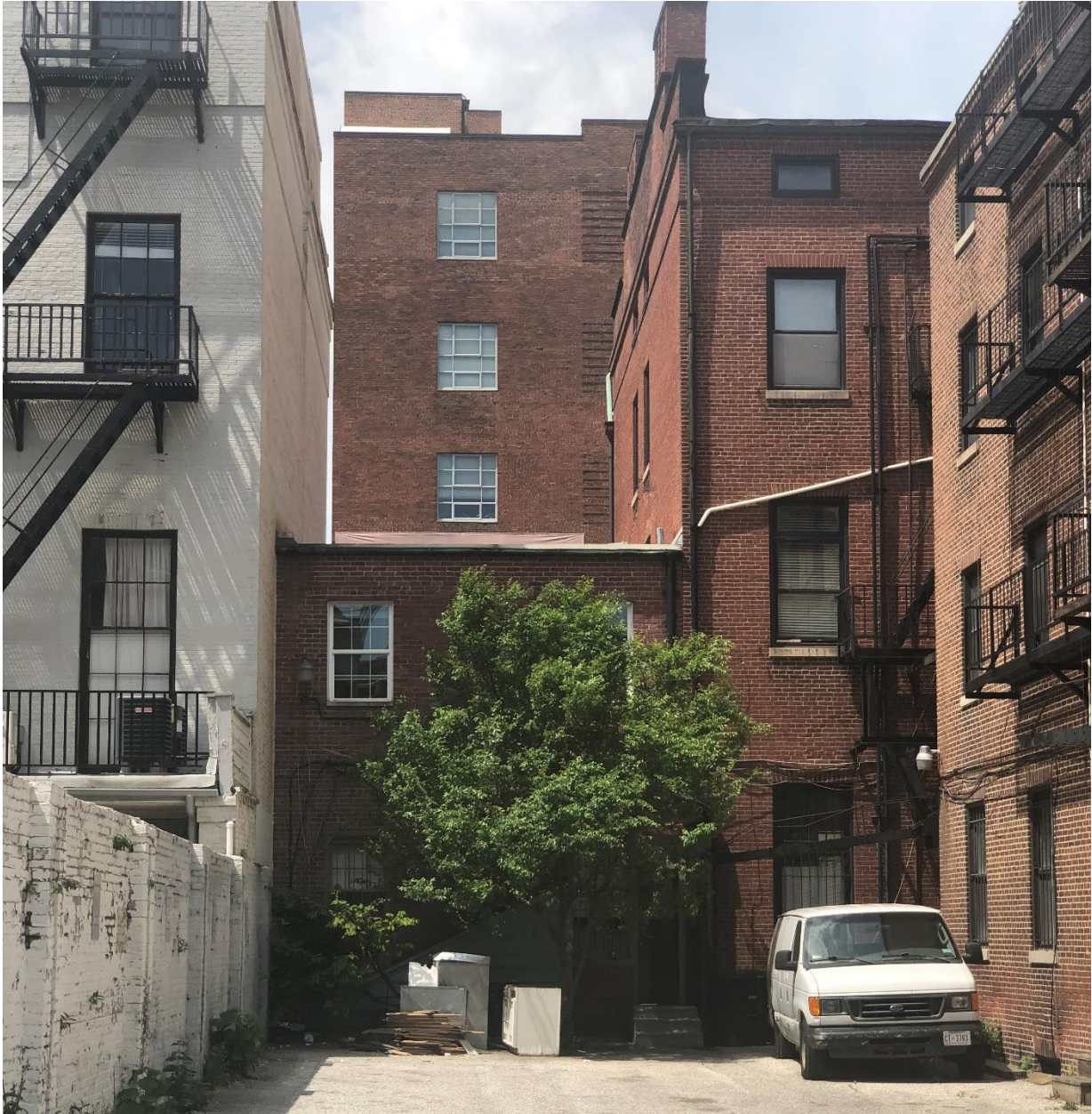
Image 2: View of rear of building
